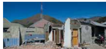
Buildings ravaged by the earthquake.
